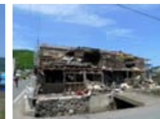
Photo 14 Heavily damaged wood-frame building
