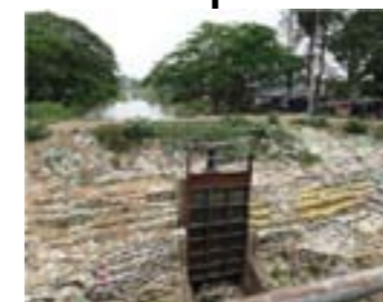
Location E A sluice gate
