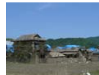
Photo 13 Scene of damage in Hojo district
