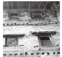
Photo 12 Cutting edge of joists exposed at floor levels
