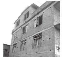
Photo 1 Masonry + RCC beams
