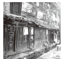
Photo 7 dalan + wooden doors
