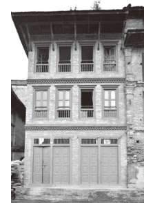
Photo 11 Cornice on different floor levels
