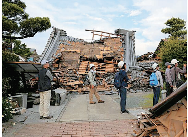
Collapsed roof of temple due to earthquake (Year: 2016, Mashiki Town, Kumamoto Prefecture)
